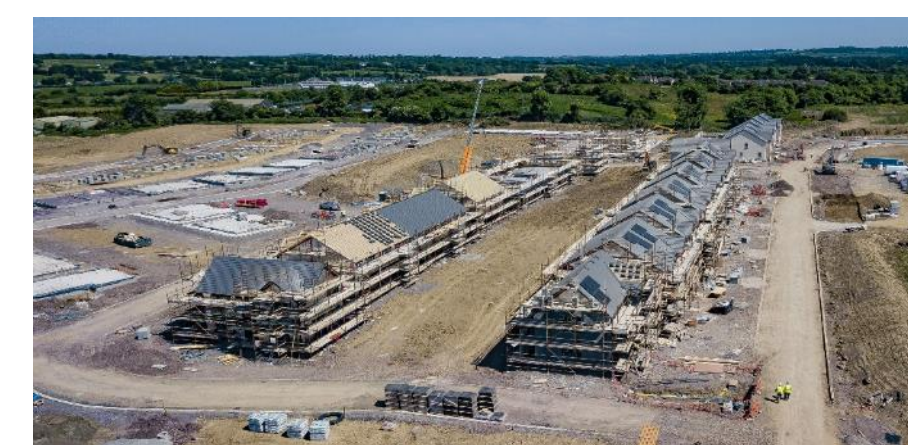
Timber frame construction at Glenveagh Cluain Adain
